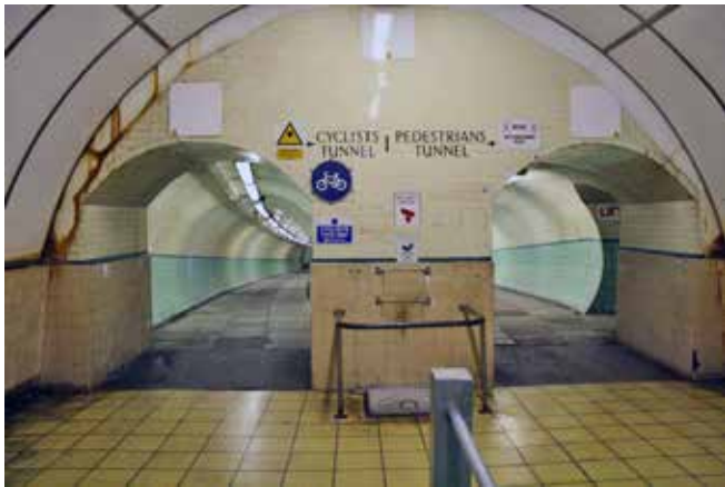
The Tyneside Tunnel in 2009.
